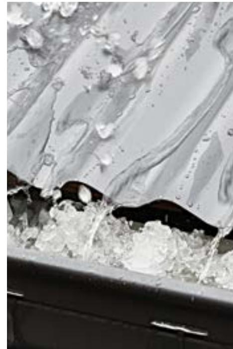
Accumulated hail in a gutter without gutter mesh installed
